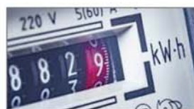
High energy consumption
